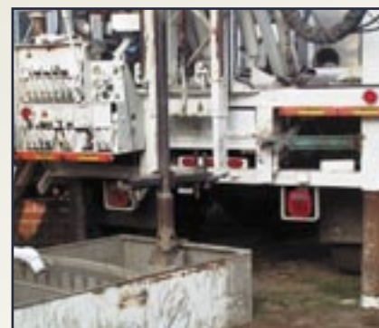
Mobile B-61 Drill Rig
