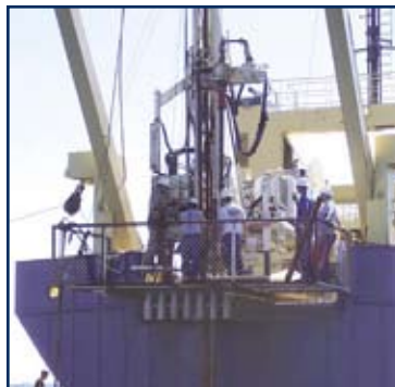
B-80 drill rig during a site investigation in the Sea of Cortez
