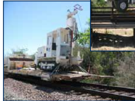
Limited access drilling on the T-Railer®
