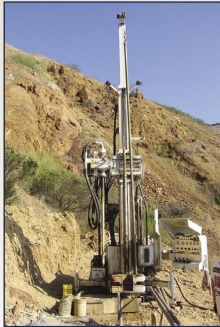
Track mounted Fraste rig working in a difficult access location.
