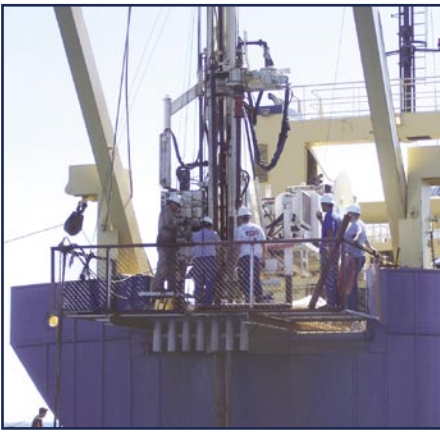
B-80 Drill rig during investigation in Puerto Libertad, Mexico.
