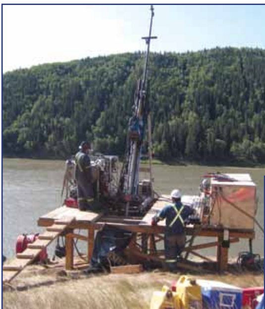
Above: Angled drilling on a slope
