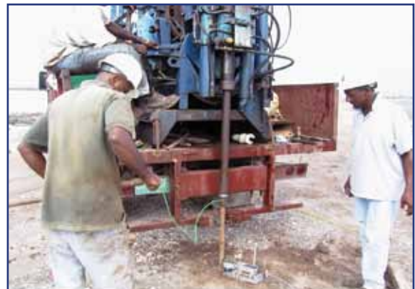
CPT Testing with Local Drill - Jamaica
