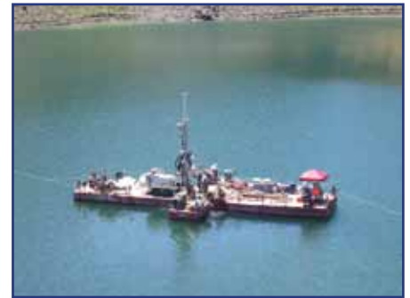
Mud Rotary Drilling & CPT - Flexifloat Sectional Barge
