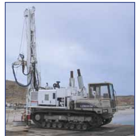
Mud Rotary Drilling at Tailings Impoundment
