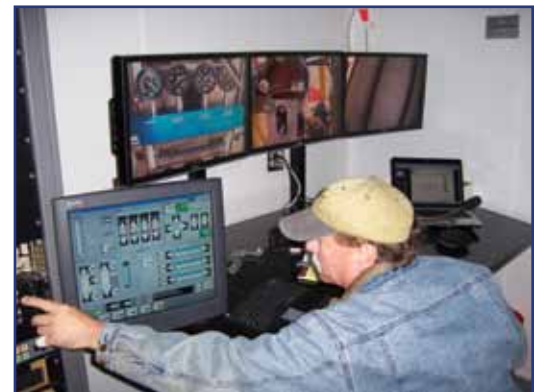
Operator inside containerized control unit.
