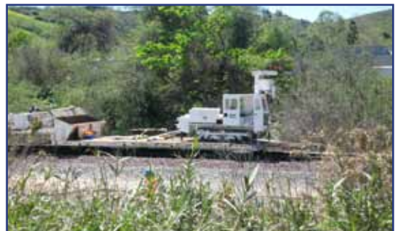
Limited access drilling on the T-Railer®
