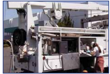
Water quality monitoring cabinet
