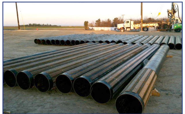
Below: Well screen and casing presented in order ready for installation.
