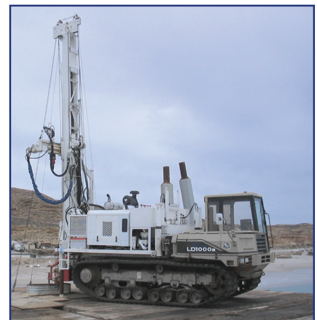
Mud Rotary Drilling at Tailings Impoundment
