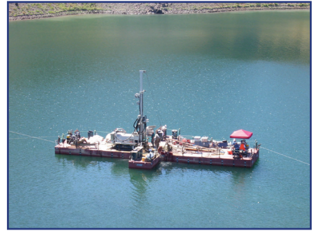
Mud Rotary Drilling & CPT - Flexifloat Sectional Barge
