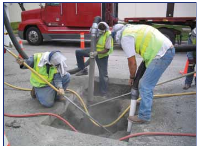
The high-pressure/high-volume air combined with the specially designed nozzle breaks up the hardest soils in record time.
