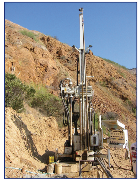
Slope Stability Investigation for Reclamation of Former Quarry Site - Track-mounted Fraste Mud Rotary Drill Rig
