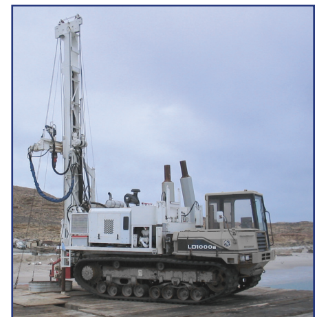
Mud Rotary Drilling at Tailings Impoundment
