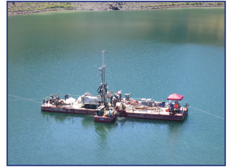
Mud Rotary Drilling & CPT - Flexifloat Sectional Barge
