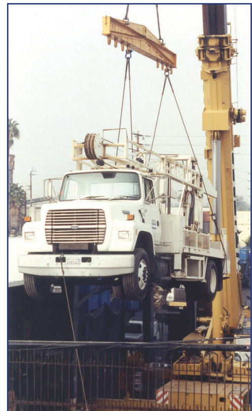
Marl M12 Drill Rig deployed by a 175 ton crane into a difficult access drill location.
