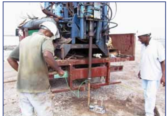
CPT Testing with Local Drill - Jamaica
